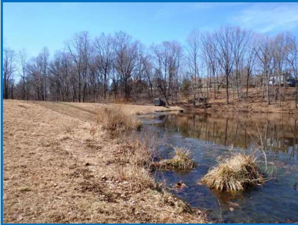
Figure 29 - Looking across upstream embankment towards right abutment
