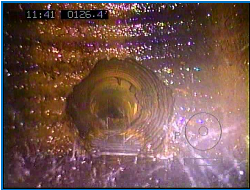
Figure 24 - Looking across riser into low level drain pipe
