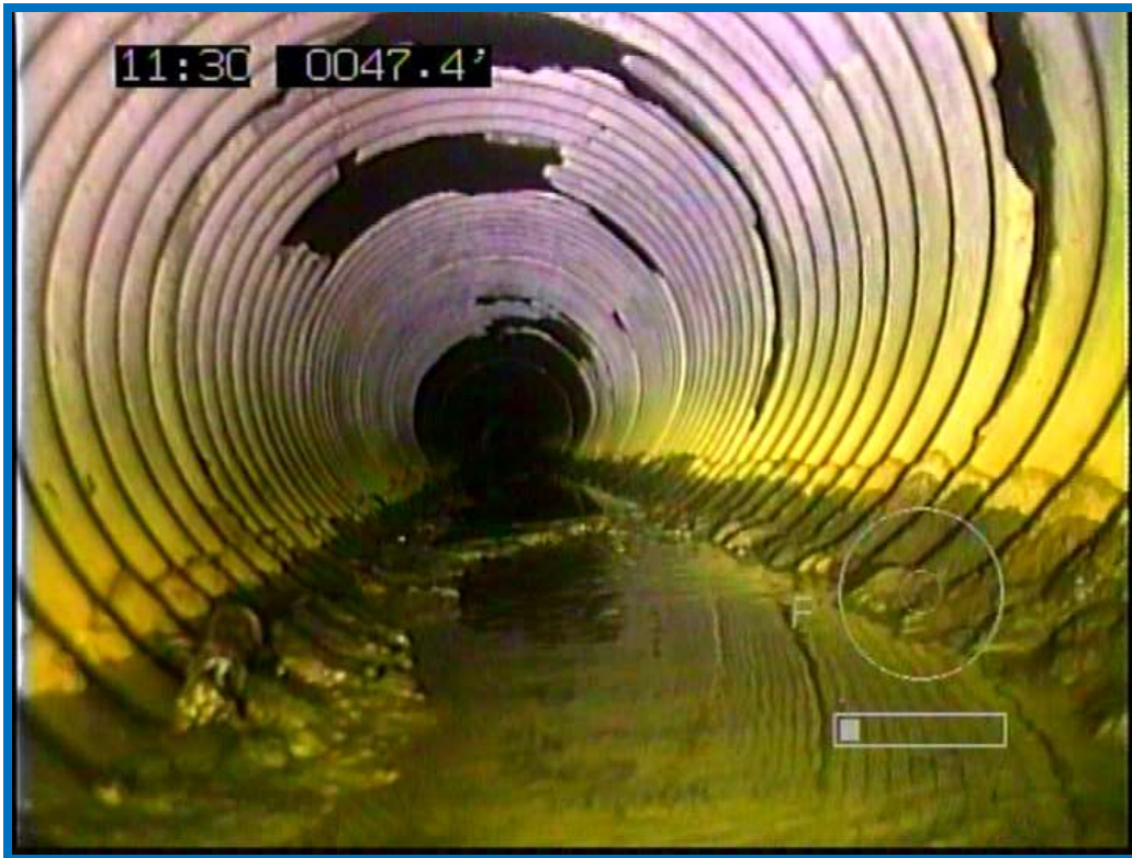
Figure 20 - Typical view of existing CMP, note patches of coating
