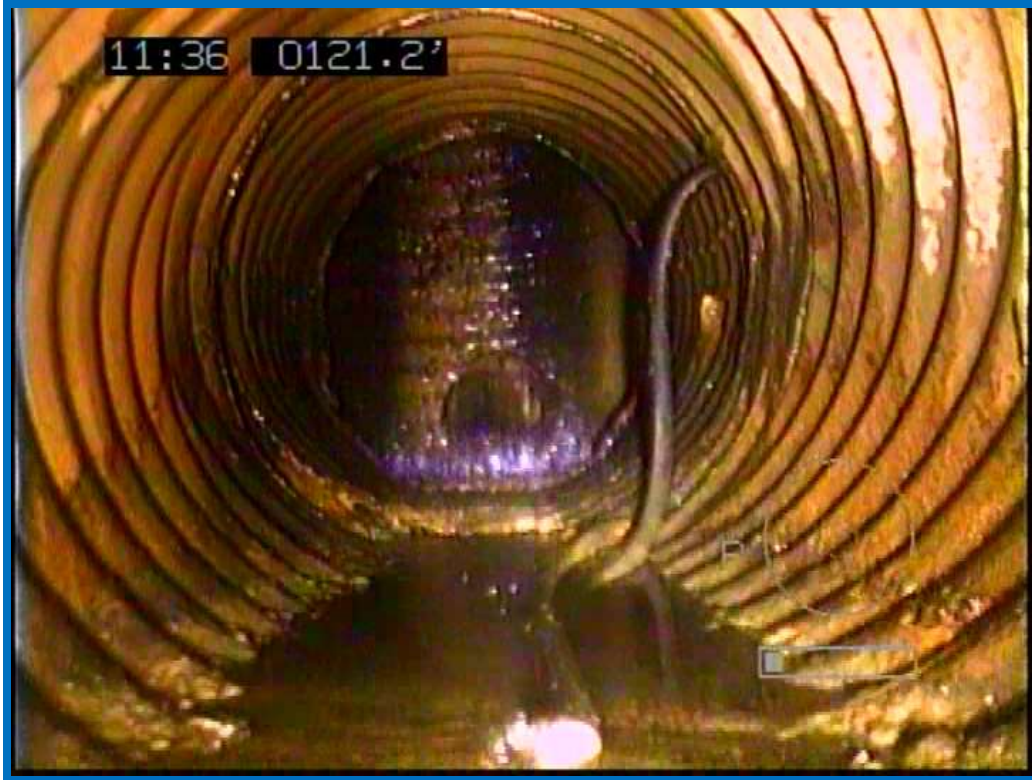
Figure 21 - Joint 7 as it transitions to riser
