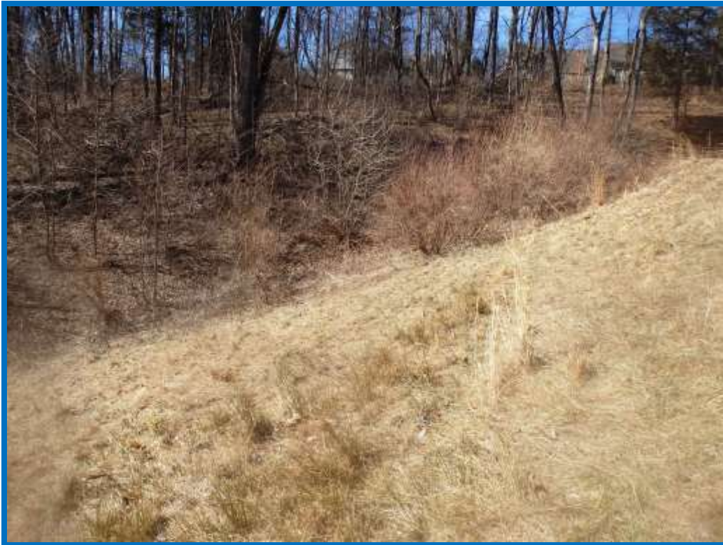
Figure 26 - Middle of the dam looking towards the right abutment
