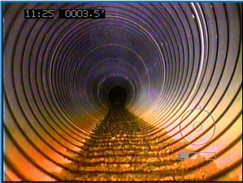
Figure 18 - Picture inside new section of CMP
