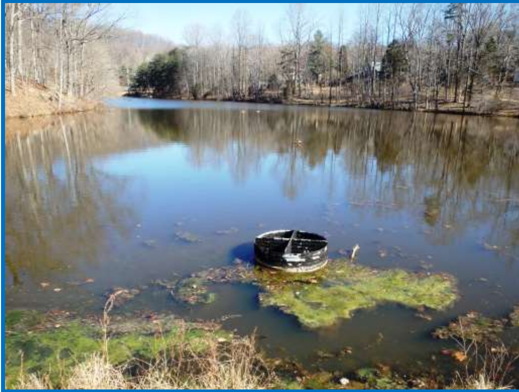
Figure 1 - Riser with Trash Rack
