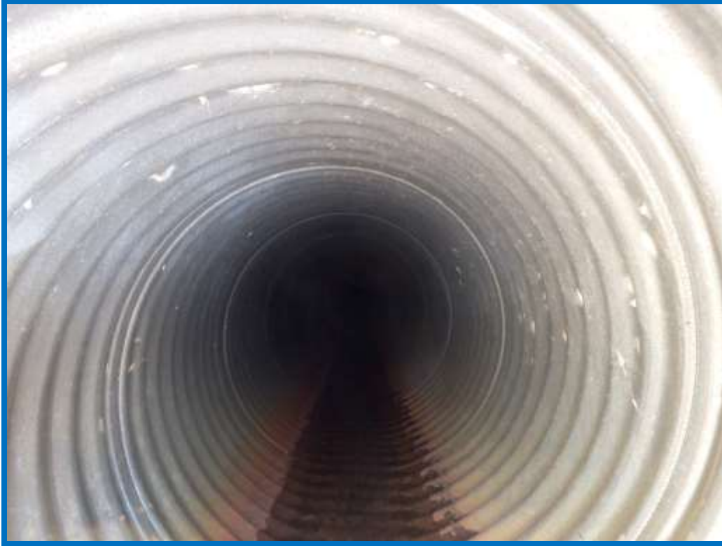
Figure 17 - Looking up into new section of CMP outfall
