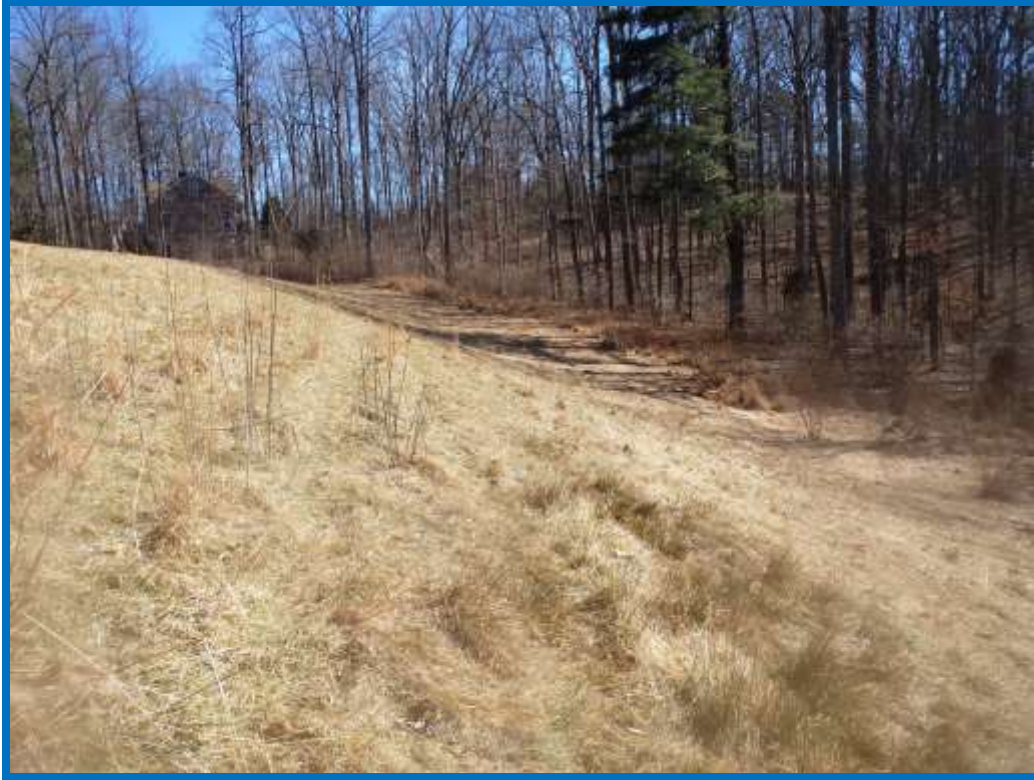
Figure 25 – Middle of the dam looking towards the left abutment
