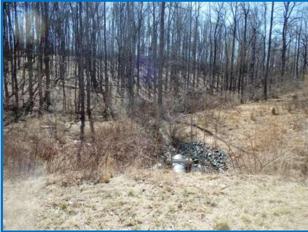
Figure 13 - Looking downstream at plunge pool and outfall pipe
