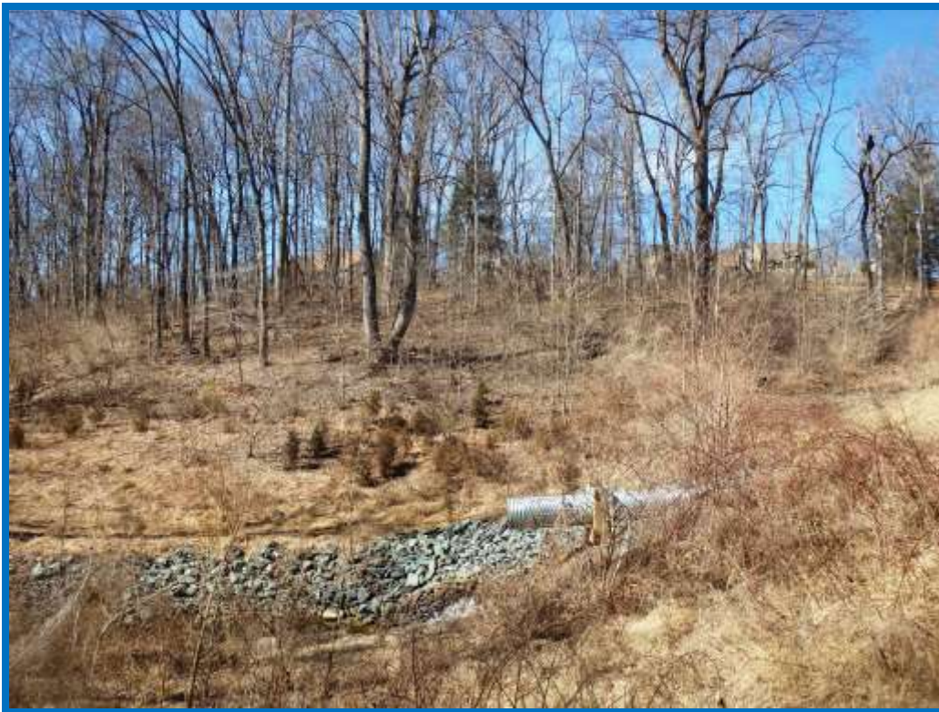
Figure 14 - Looking towards right abutment at primary spillway outfall pipe
