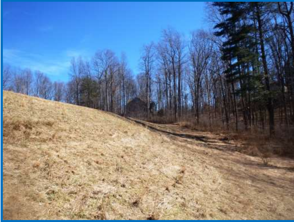
Figure 27 - Auxiliary Spillway and channel
