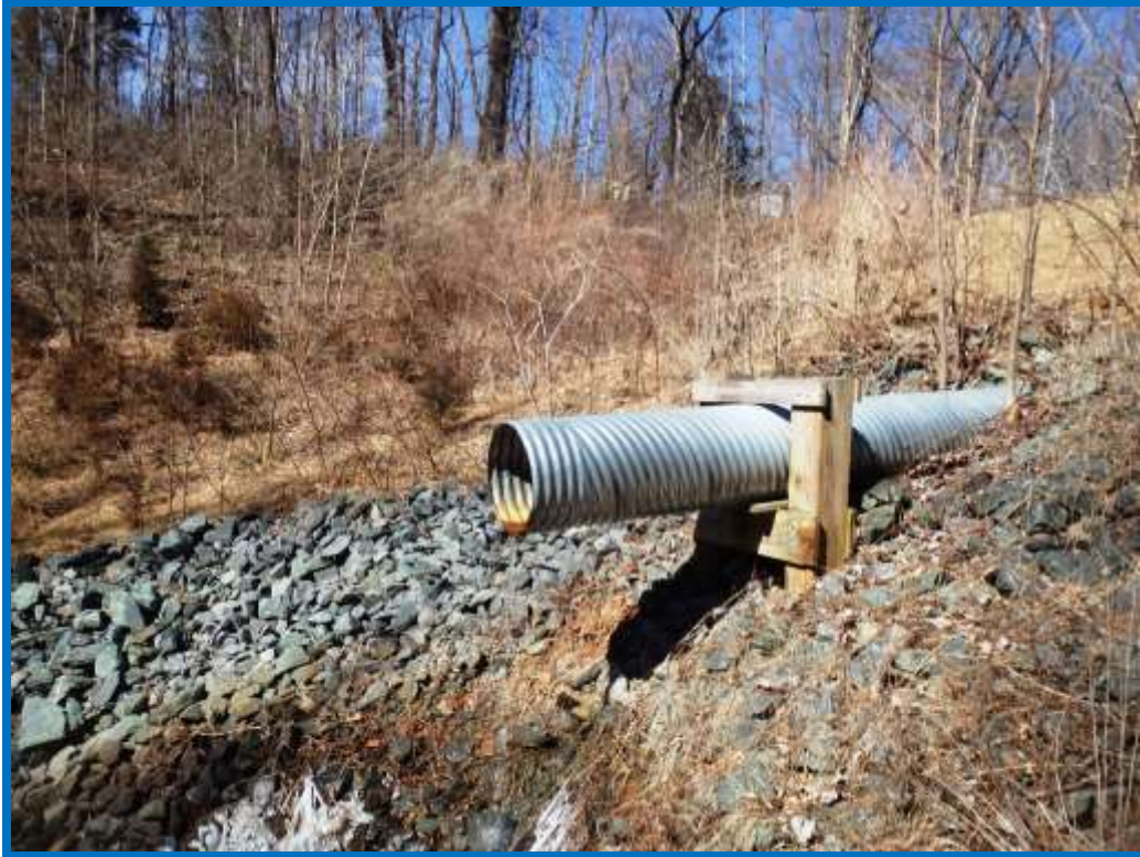
Figure 15 - Outfall Pipe and support
